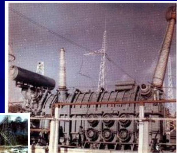
Autotransformer for 1150kV
