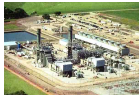
Figure : Gas plant
