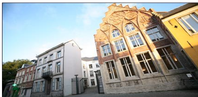
Faculty of Economics and Business Campus Leuven - Restored historical facade
